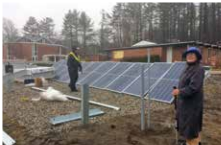
A rainy-day picture of Trudy Richter Mott-Smith '52 and the un-installed solar panels to be used in the solar array.
